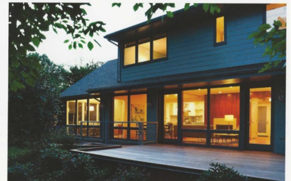
The rear deck is only 14 inches above the ground and is edged with a wheel stop instead of a railing.
